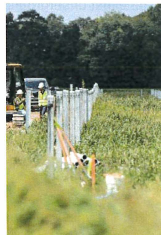
Figure 3. Driven Piles
